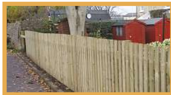
■ The new fencing at Walton Road
