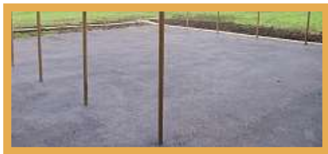
■ The newly tarmaced drying area
