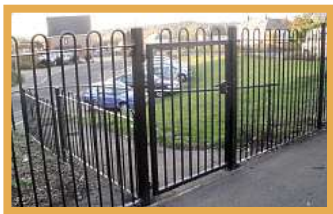
■ The new security gates in place
