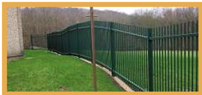
■ The new fencing in place
