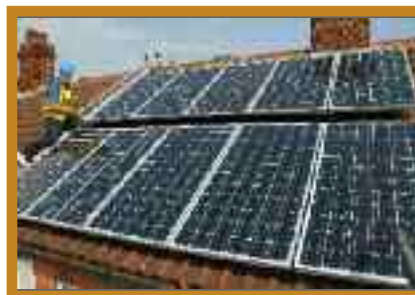
■ Installing the panels
