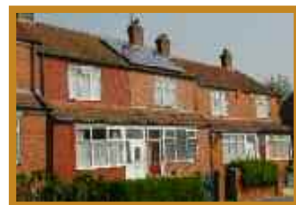
■ View of the solar panels.
